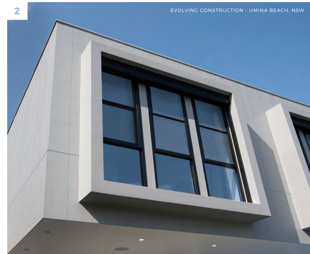
2 PROJECTING WINDOW FRAMES MAKE A GREAT FEATURE EVOLVING CONSTRUCTION - UMINA BEACH, NSW
