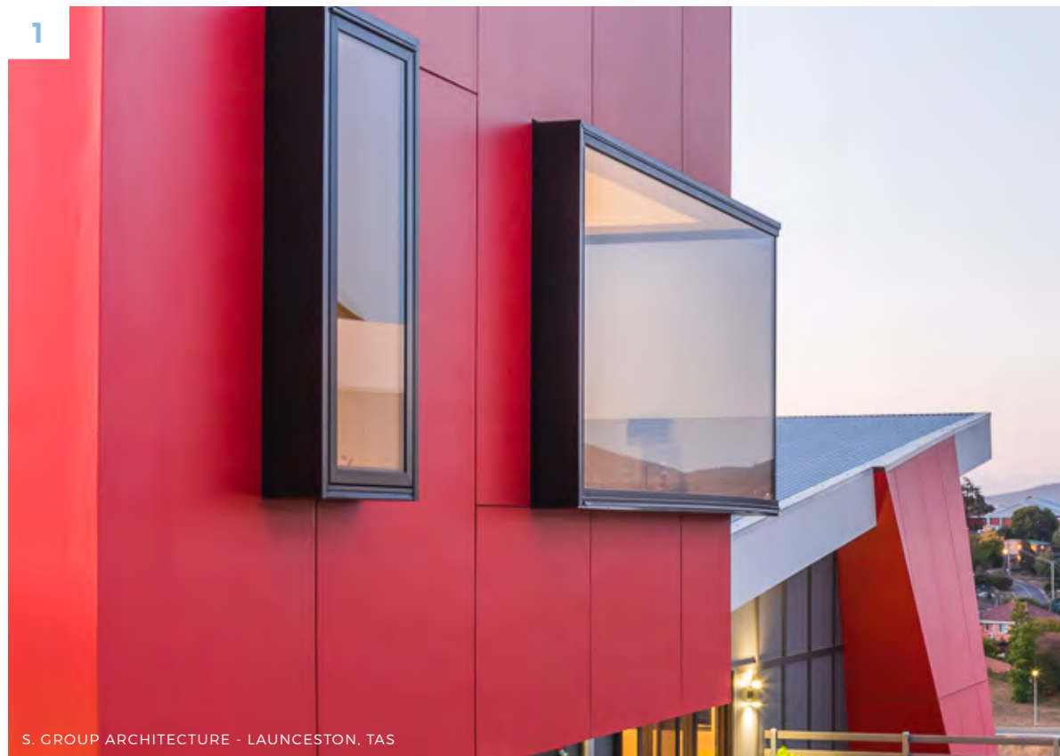
1 ORIEL WINDOW IN S GROUP ARCHITECTURE'S WILD BULLDOG HOUSE S. GROUP ARCHITECTURE - LAUNCESTON, TAS
