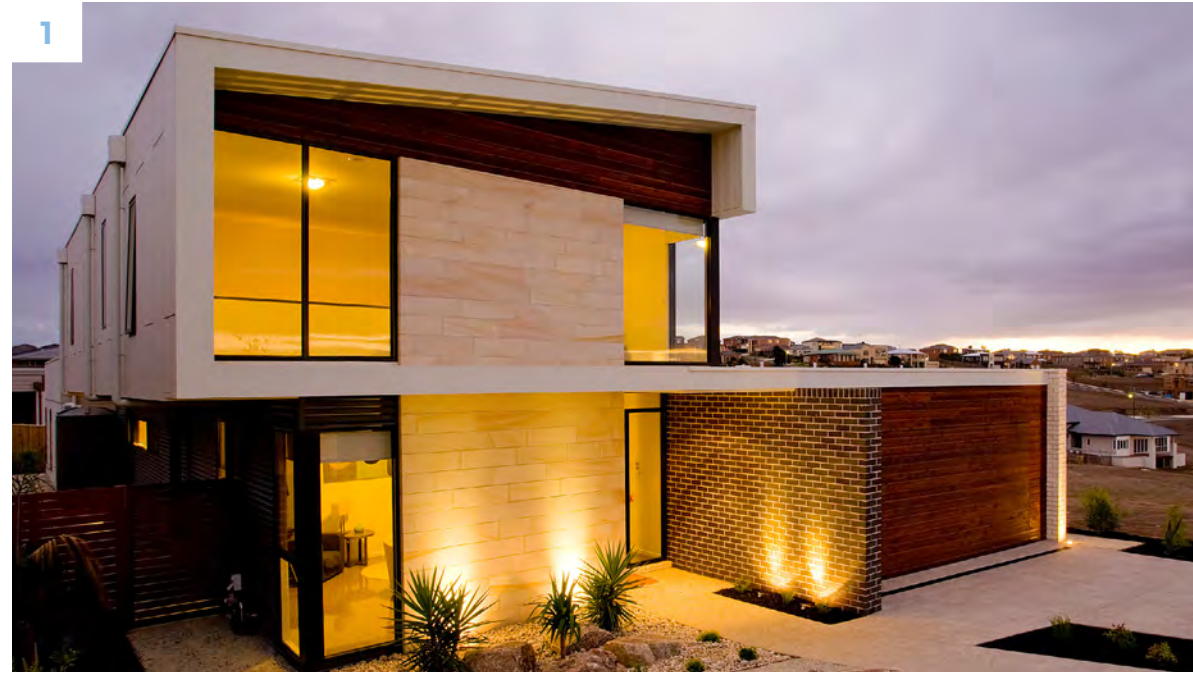
1 A MIX OF BRICK, STONE, TIMBER AND MATRIX™ CLADDING
