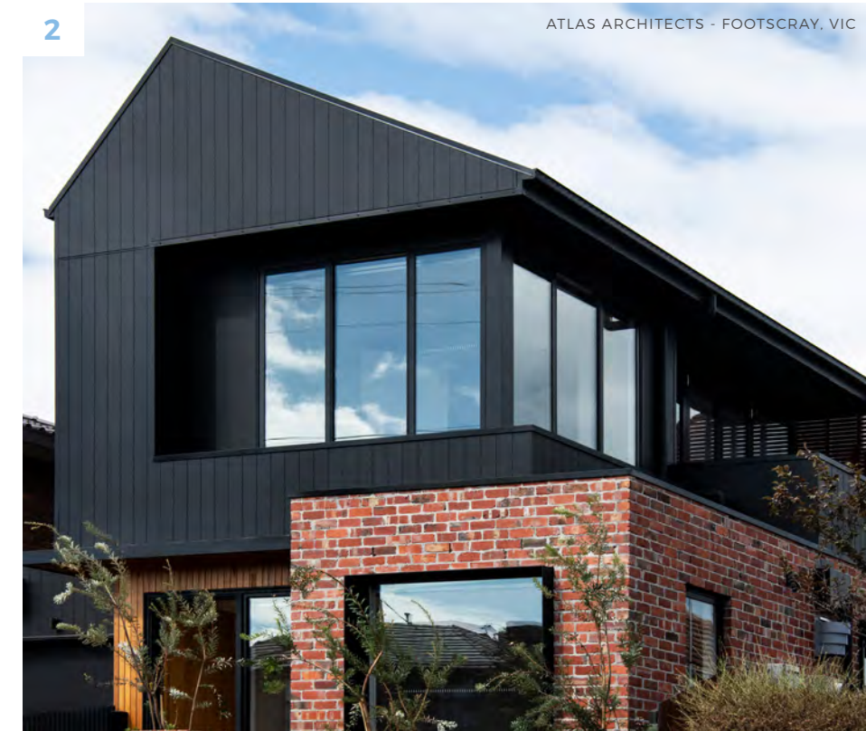
AN ASYMMETRICAL SALT BOX ROOF
