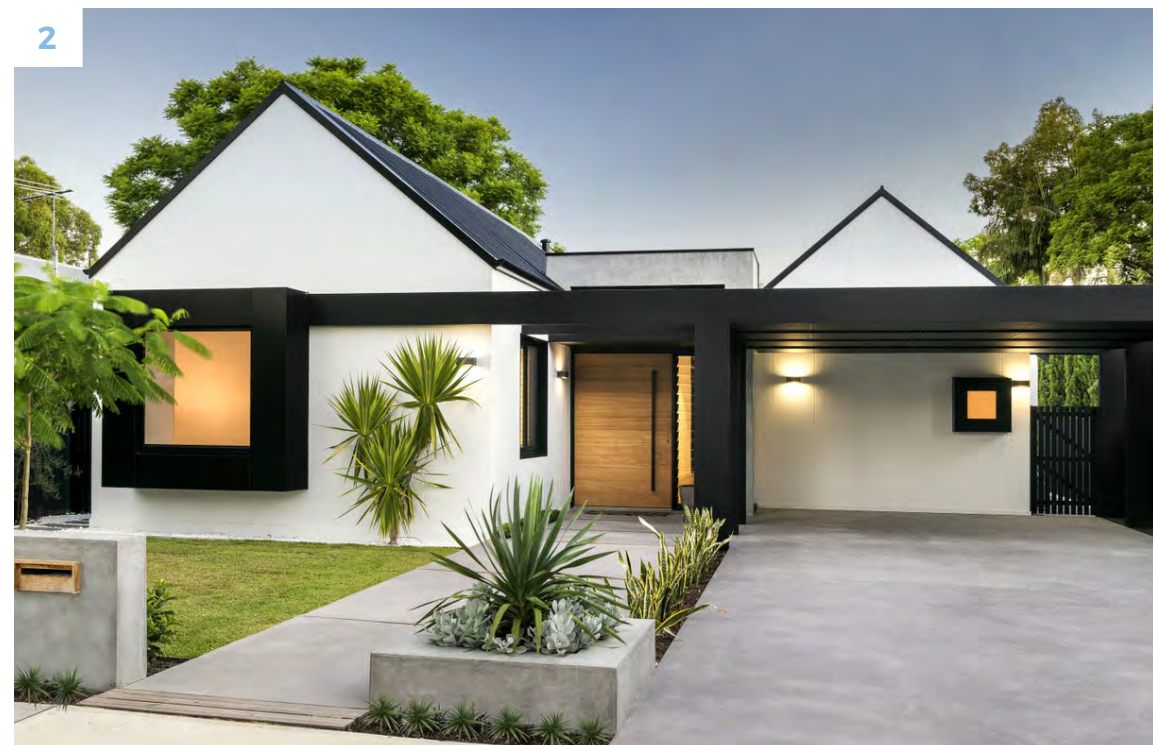
DRAMATIC WHITE AXON™ CLADDING WITH BLACK TRIMS BY MAEK BUILDERS, WA
